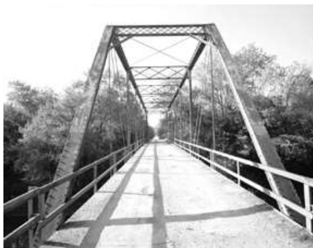
Historic Caton Ford Bridge ~ Built 1894
