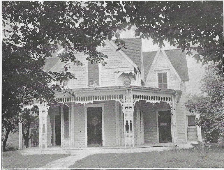
Residence of J. W. Frye
