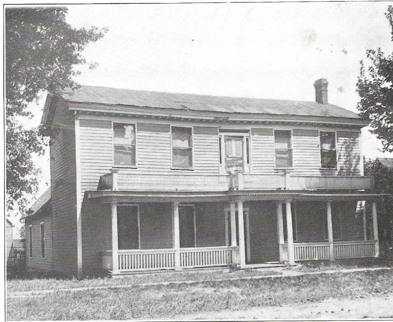
Residence of H. C. Hickman—County Recorder
