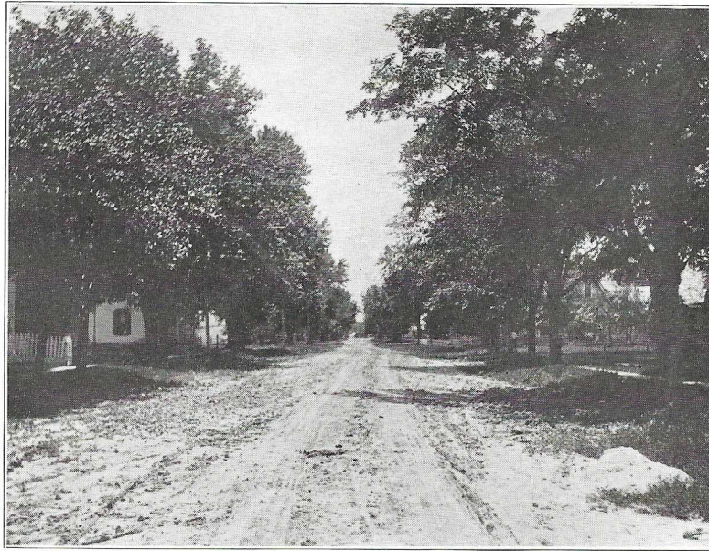
North Washington street, looking south
