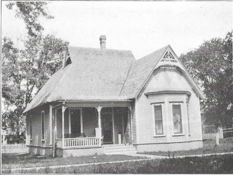
Residence of E. M. Damrell
