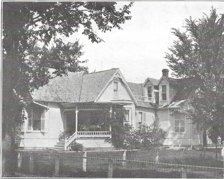
Residence of A. H. Davison
