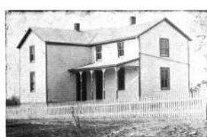
TOWN RESIDENCE OF GEO. J. CASTROP, FREEBURG, MISSOURI.
