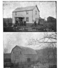
RESIDENCE AND BARN OF LEWIS FRANCIS, BYRON, MISSOURI.
