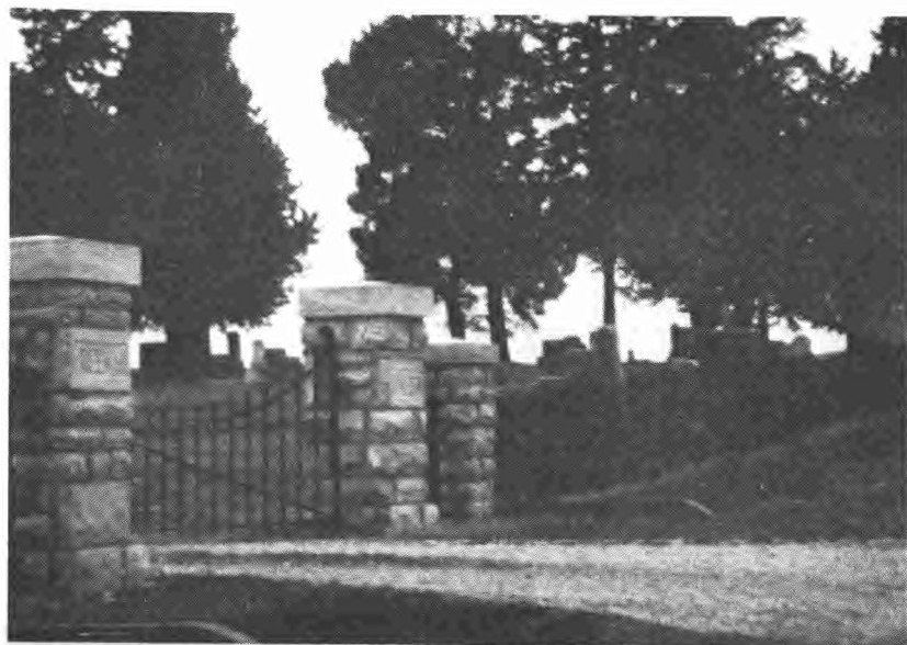
East gate and iron fence at Freeman Cemetery.
