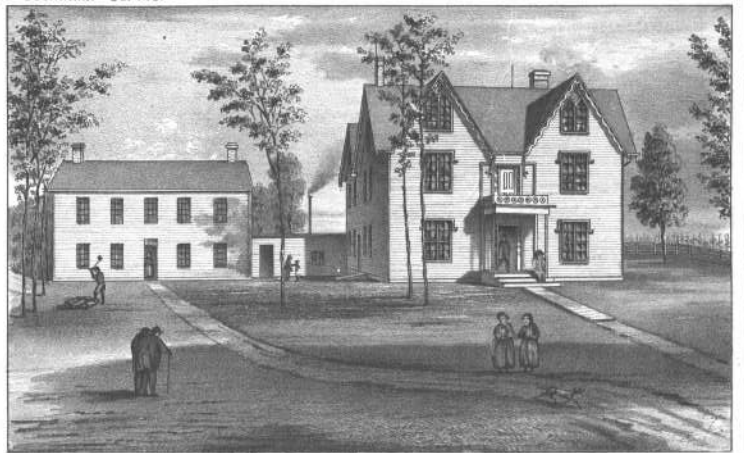
COUNTY POOR FARM BUILDINGS BUCHANAN Co. Mo.
